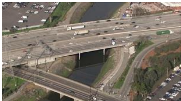
US 110 Bridge over Dominguez Channel, Los Angeles, California
