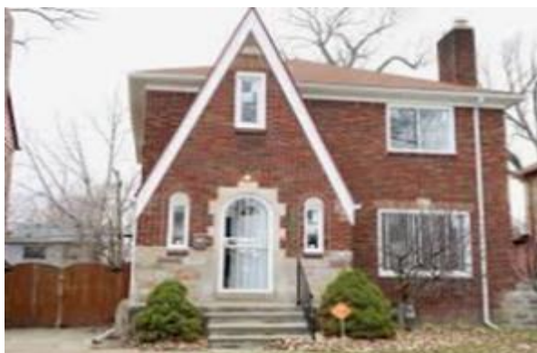
Rehabbed and Ready buildingdetroit.org
